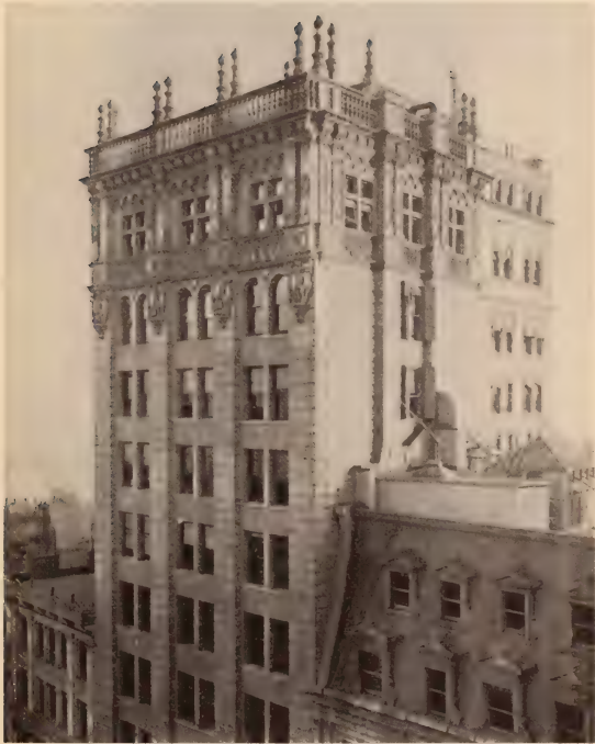
UPPER STORIES OF SAMPSON BUILDING.
